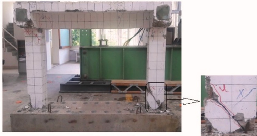
Figure 3.19: Crack pattern of the frame
