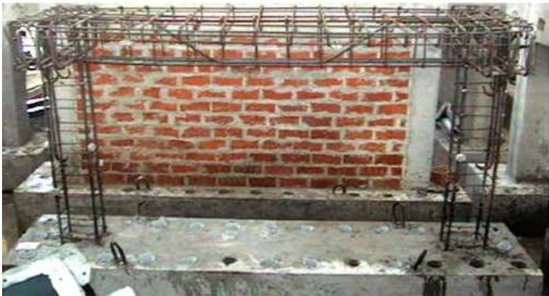
Figure 3.4: The details of frame reinforcement
