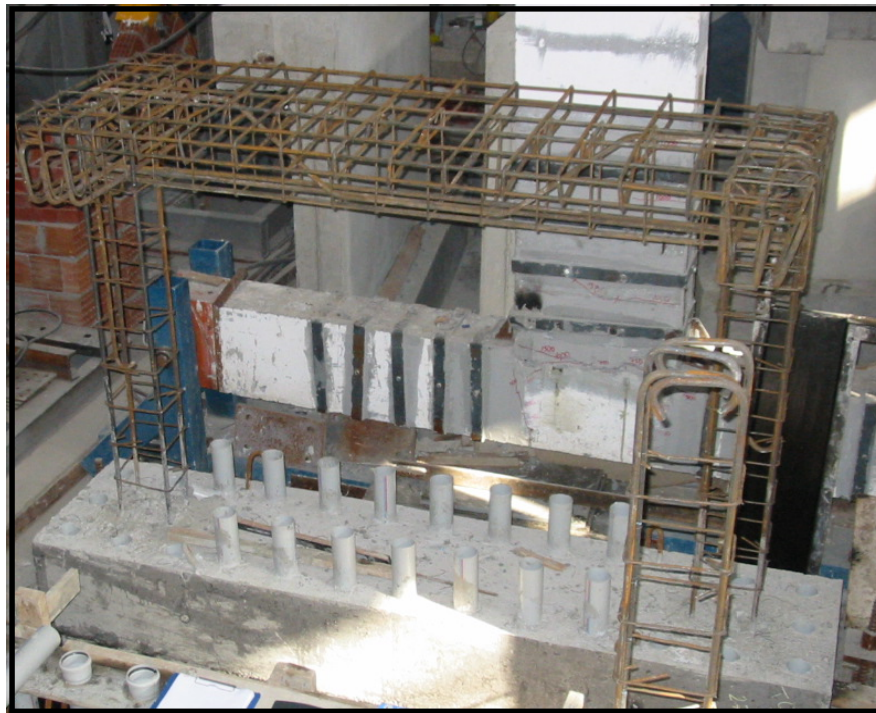
Figure 4.1: General view of preparation of the RC frame specimens at I.T.U. Laboratory.
