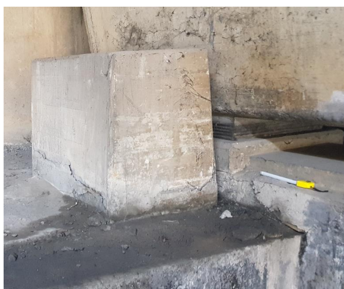
Figure 8.18. Shear Deformations at Shear Keys of Molla Gürani Viaduct
