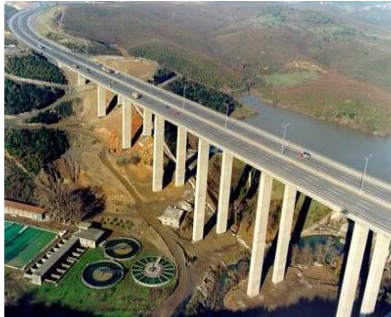
Figure 4. 2 Molla Gürani Viaduct
