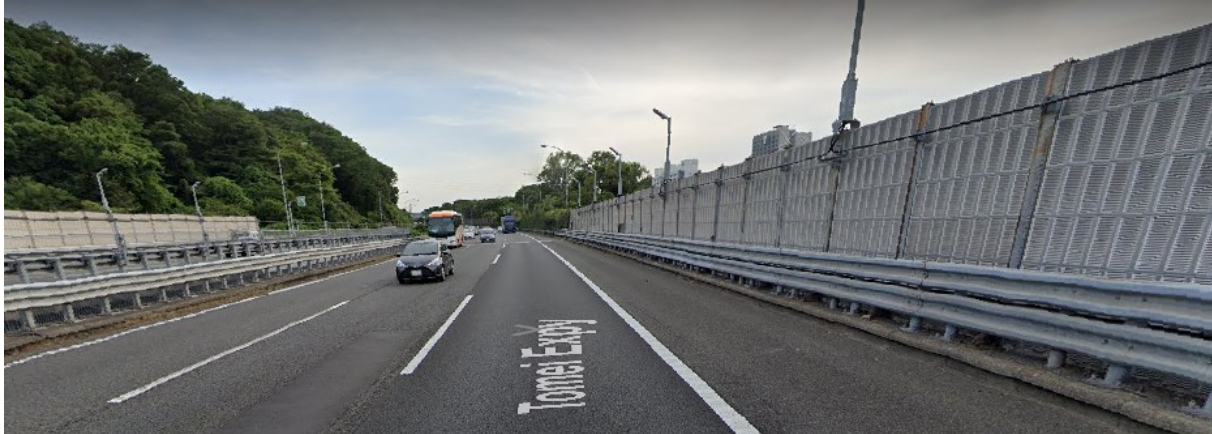
Figure 1. A noise barrier along Tomei Expressway around Yokohama [Maps Google Image]
