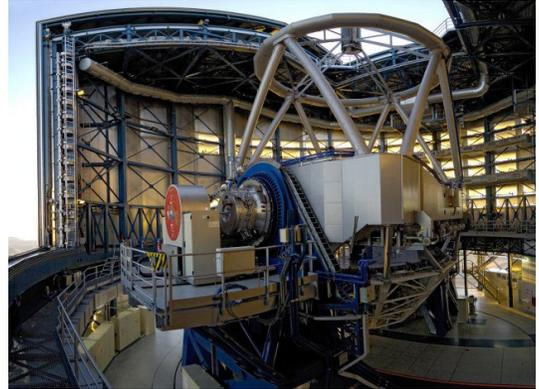
FIGURE 2. Very Large Telescope Nasmyth platform with instrumentation (Image ESO).
