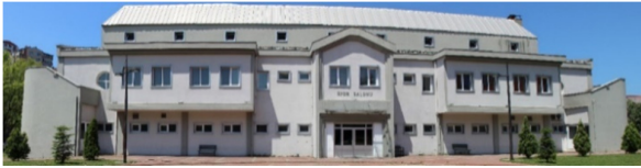
Figure 5. The selected building façade for 3D surface mesh reconstruction.
